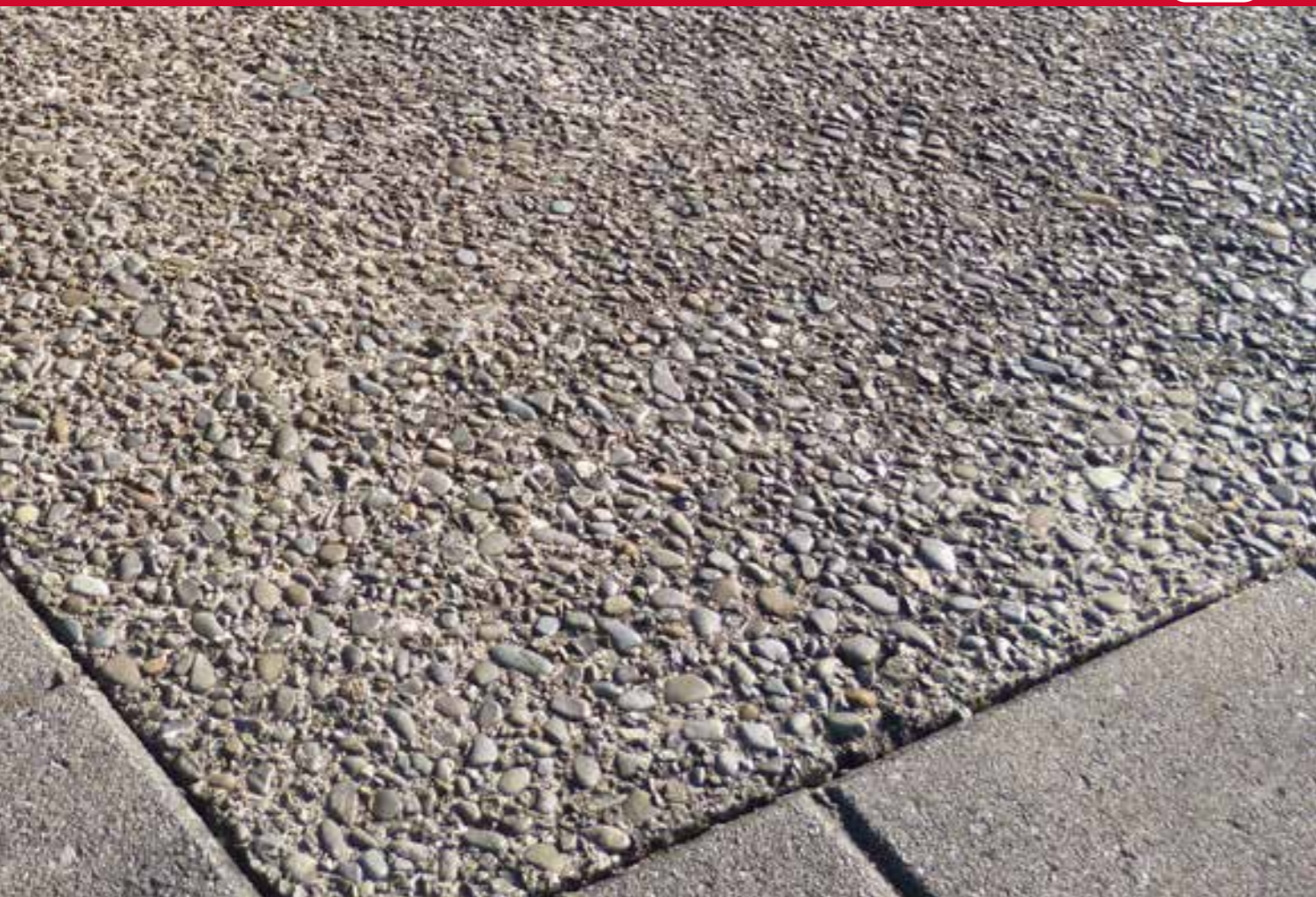
An exposed aggregate finish reveals the aggregate, resulting in an attractive, low-maintenance and slip-resistant surface
