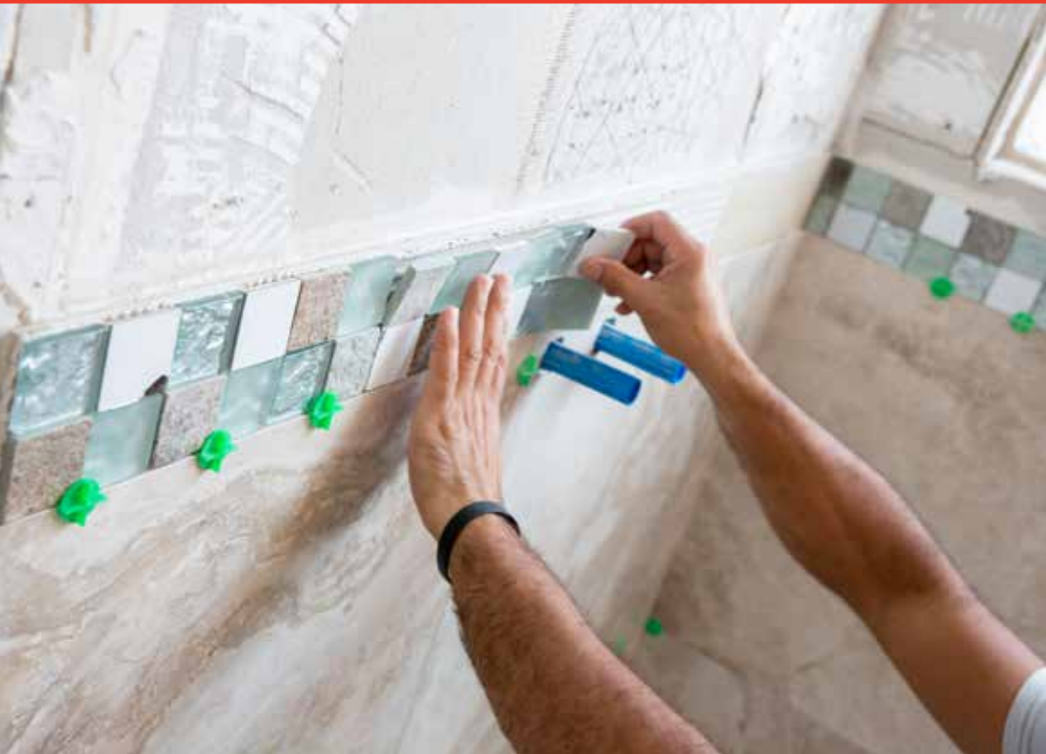
When tiling walls, remember to apply sealant around fittings and taps where they penetrate the substrate
