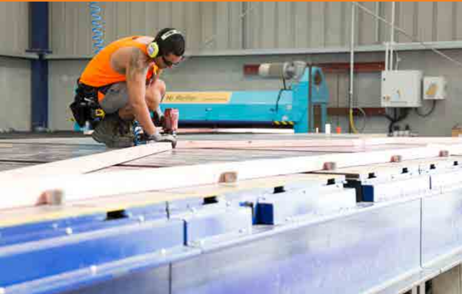
One of Steve's 70-strong team tacking trusses on the new truss bed
