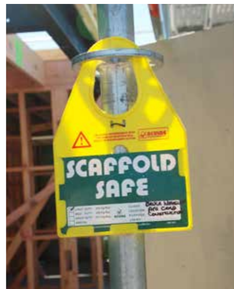
Making sure to correctly tag scaffolding is one of a number of changes that Glenn and his team at Properly Plastered have made to their health and safety plans, following a near-death accident
