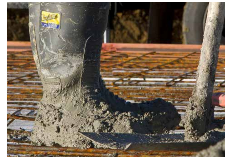
Wet cement can cause burns, if trapped against the skin. Personal protective clothing or equipment such as gloves or boots must not allow wet cement to be held against the skin
