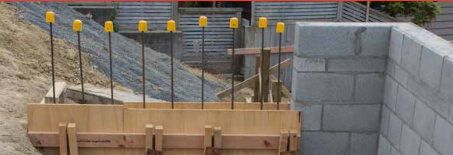
Foundation walls are straightforward to build and design on flat sites, but can be more complex when the site has uneven or sloping ground
