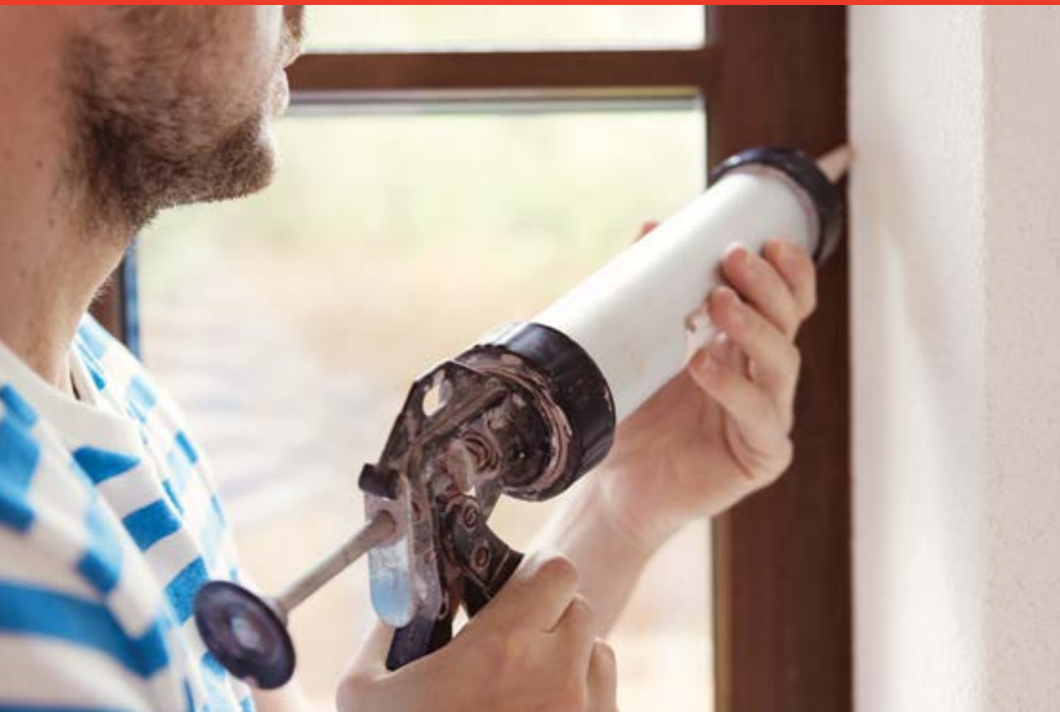
Push the sealant into the gap, moving the sealant gun forwards over the extruded sealant – do not pull the sealant gun
