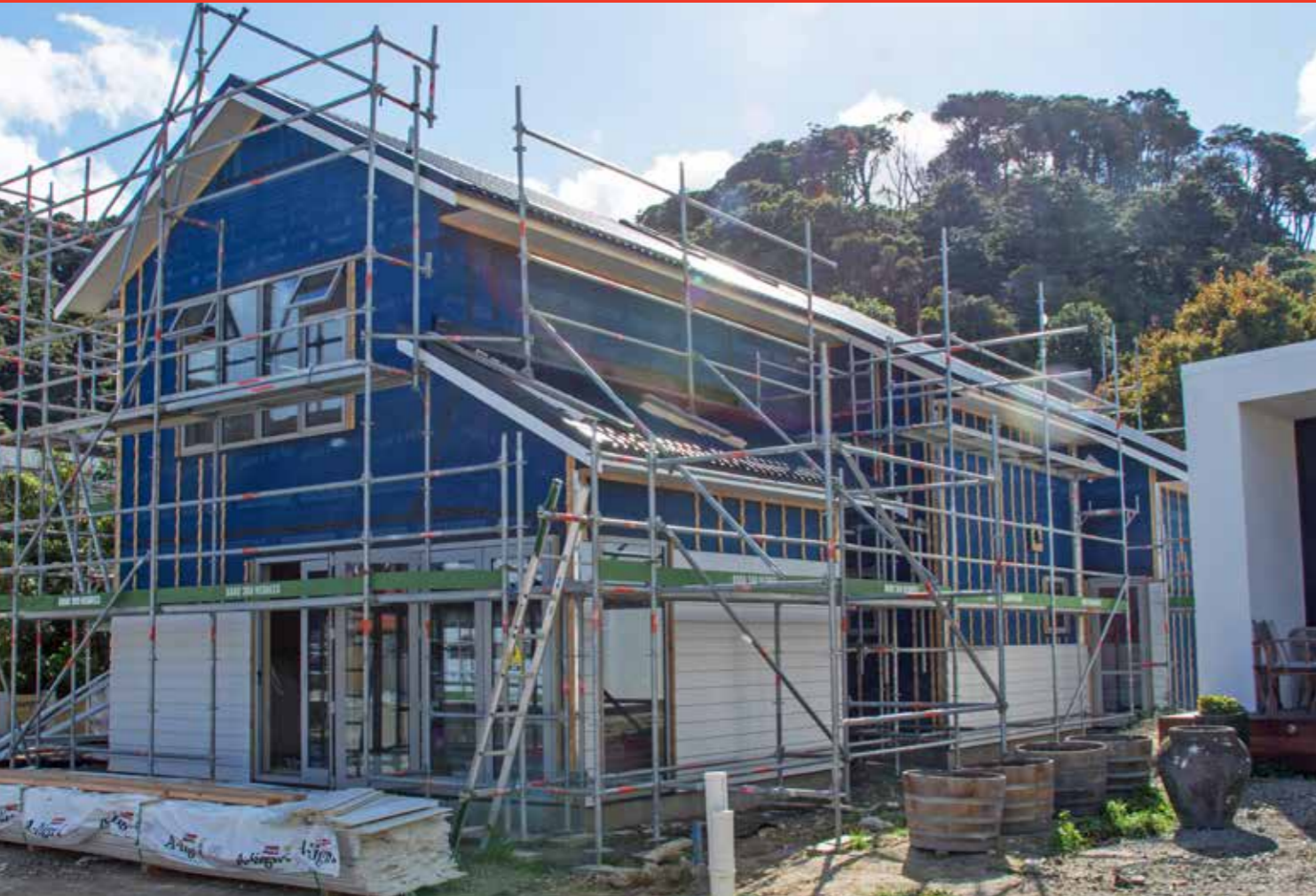
The traditional way to construct eave and verge details is to install soffit linings before the external cladding; however, this compounds the weathertightness problem. A better way to achieve a weathertight detail is to install weatherboards first.
