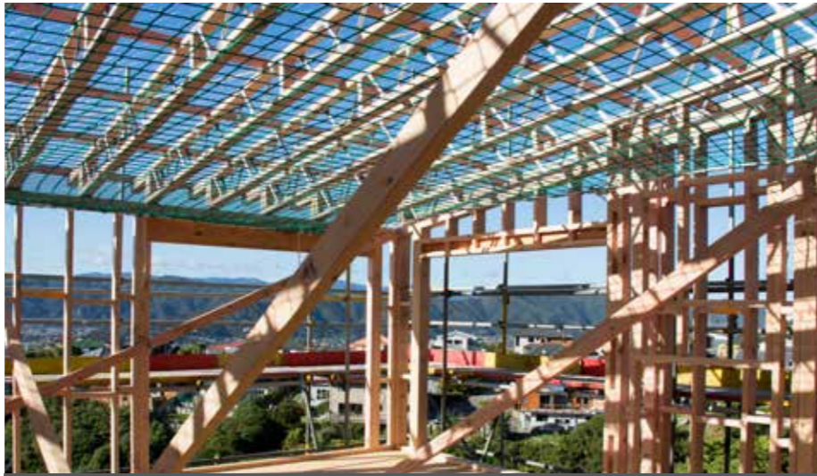
Using scaffolding and safety nets when working at height is considered best practice, but that doesn’t mean it’s reasonably practicable for every situation
