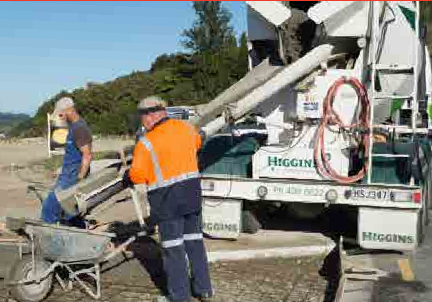
The full discharge of concrete from ready-mix trucks should be completed within 90 minutes after the commencement of mixing
