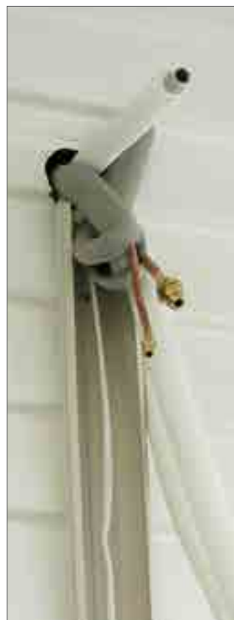
Figure 3a: Hoses coming through the top of the exterior wall
