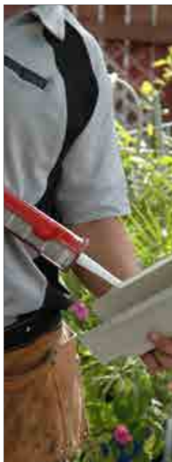
Figure 3c: Applying sealant to cover
