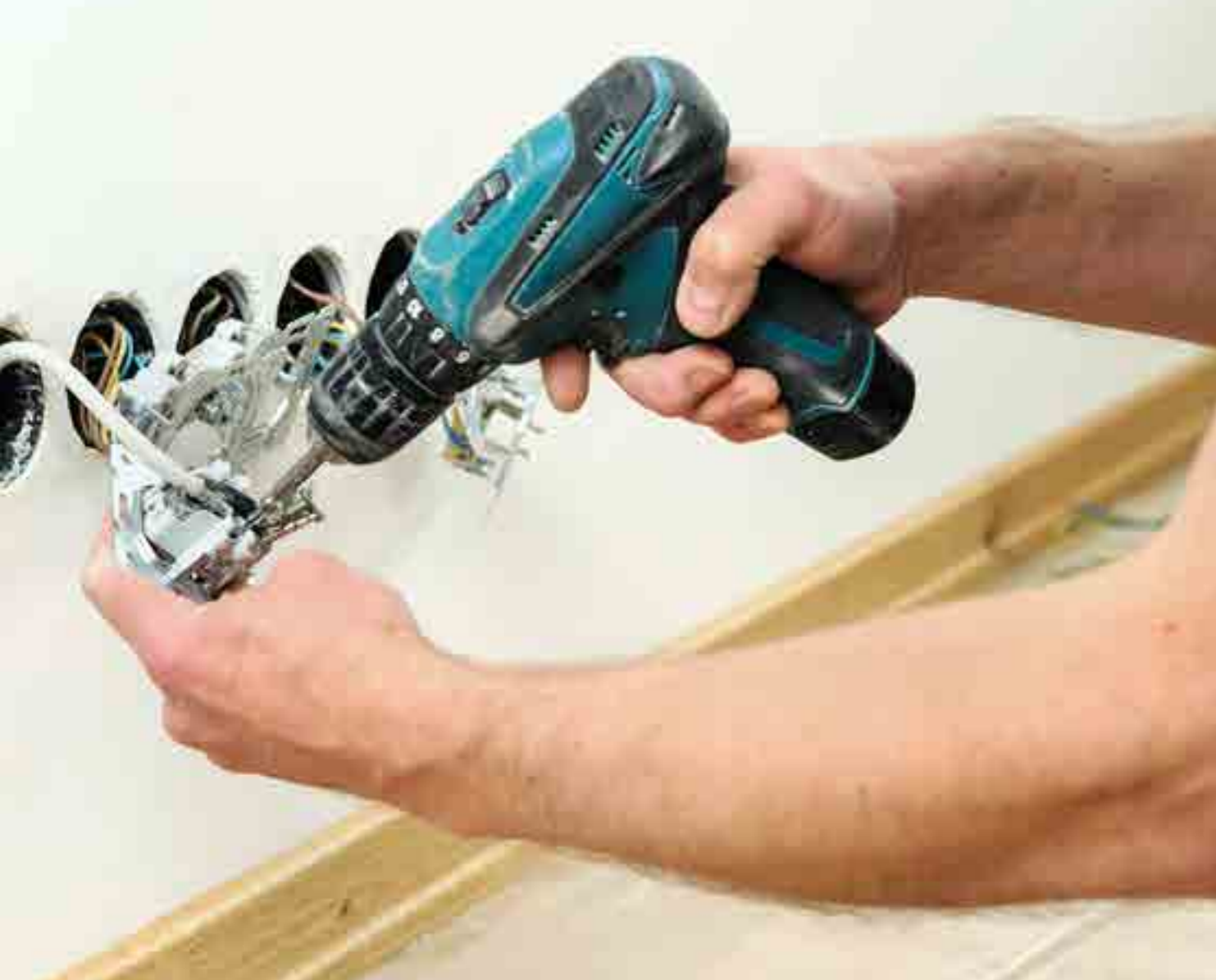
Occasionally a penetration may need to be made through an existing wall cladding, such as when installing new TV, phone or data cabling
