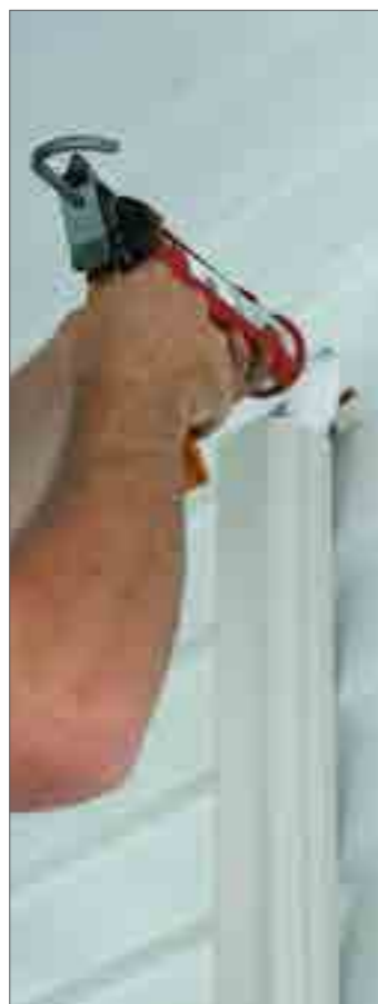
Figure 3b: Applying sealant around pipework
