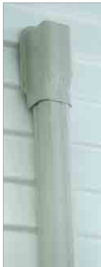
Figure 3d: Cover in place over penetration and fully sealed to cladding
