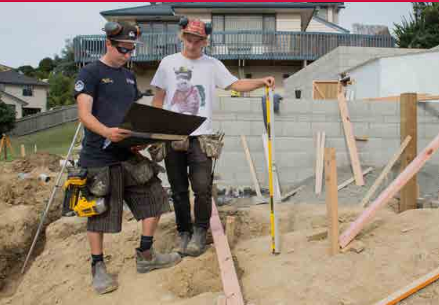
Supervision mostly involves direct site contact with co-workers and observation of the building work taking place
