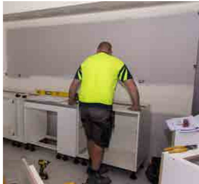
PlaceMakers SFI Kitchens service includes kitchen design, fabrication, delivery, installation and a post-installation quality check
