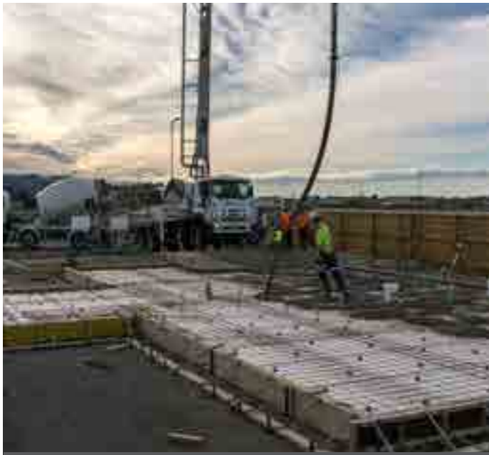
PlaceMakers SFI Foundations service includes site preparation, piping and plumbing, concrete placing and management of all council inspections and engineer checks throughout the process
