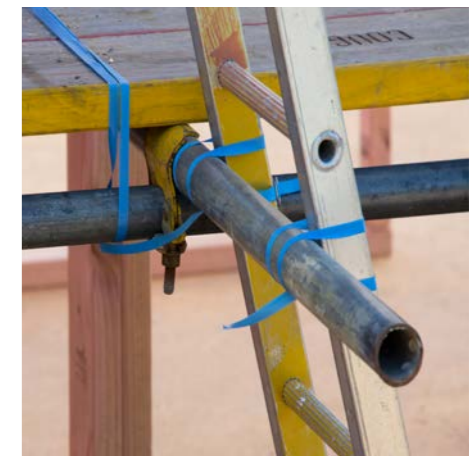
You should secure the top and bottom of ladders to prevent them from slipping sideways or falling backwards
