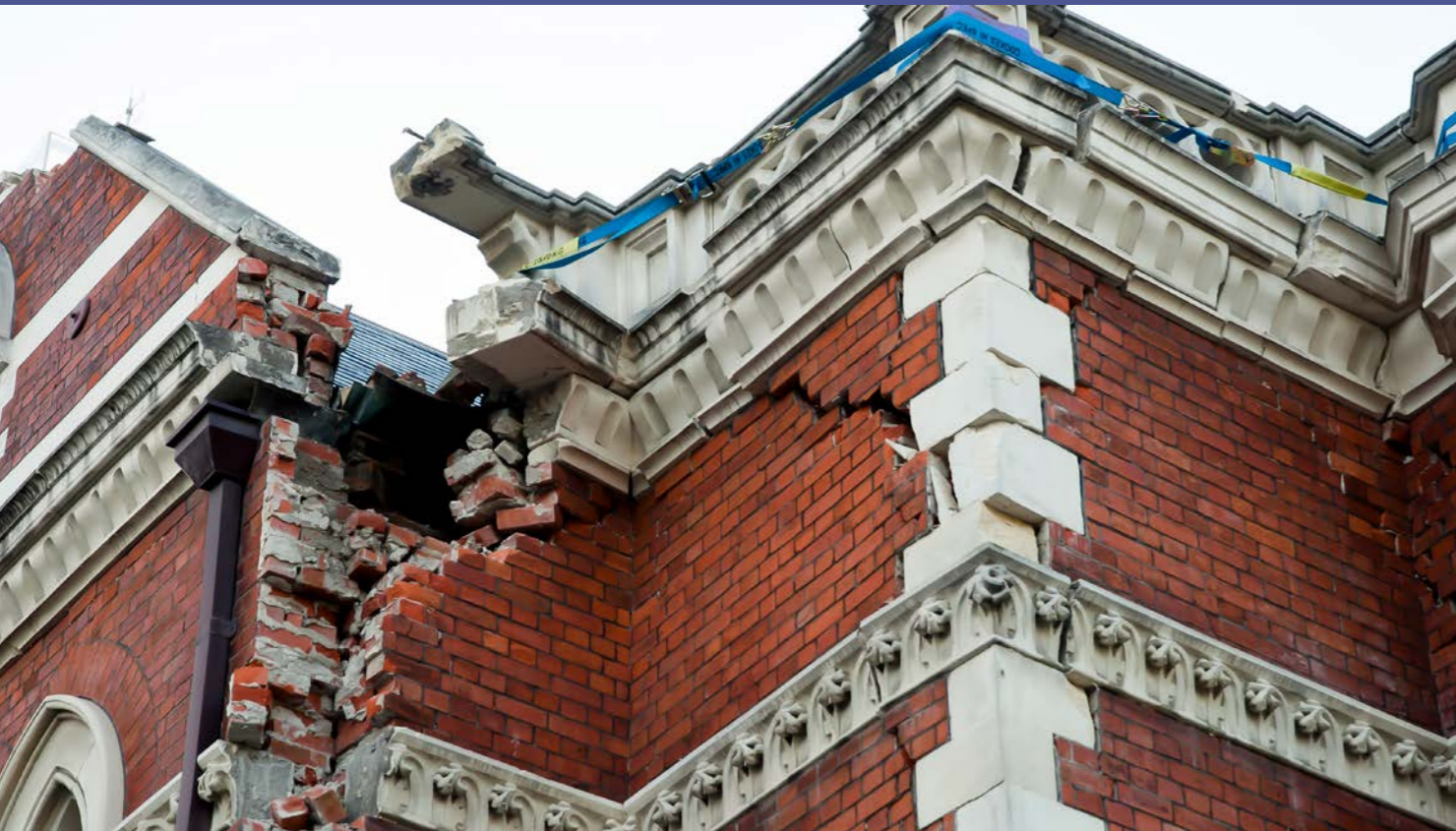
Defining earthquake-prone buildings and their associated level of risk has been a focus of MBIE since the Christchurch earthquakes
