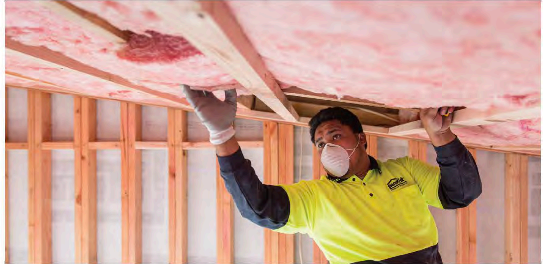
The benefits of adequate home insulation extend well beyond comfort
