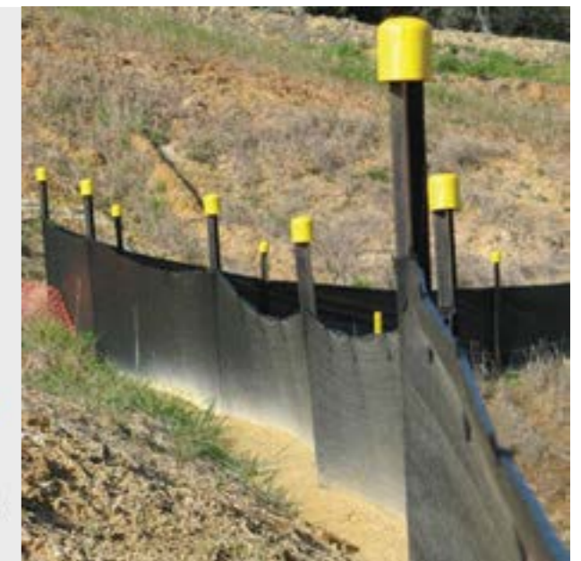
A silt fence reduces sediment run-off on sloping sites
