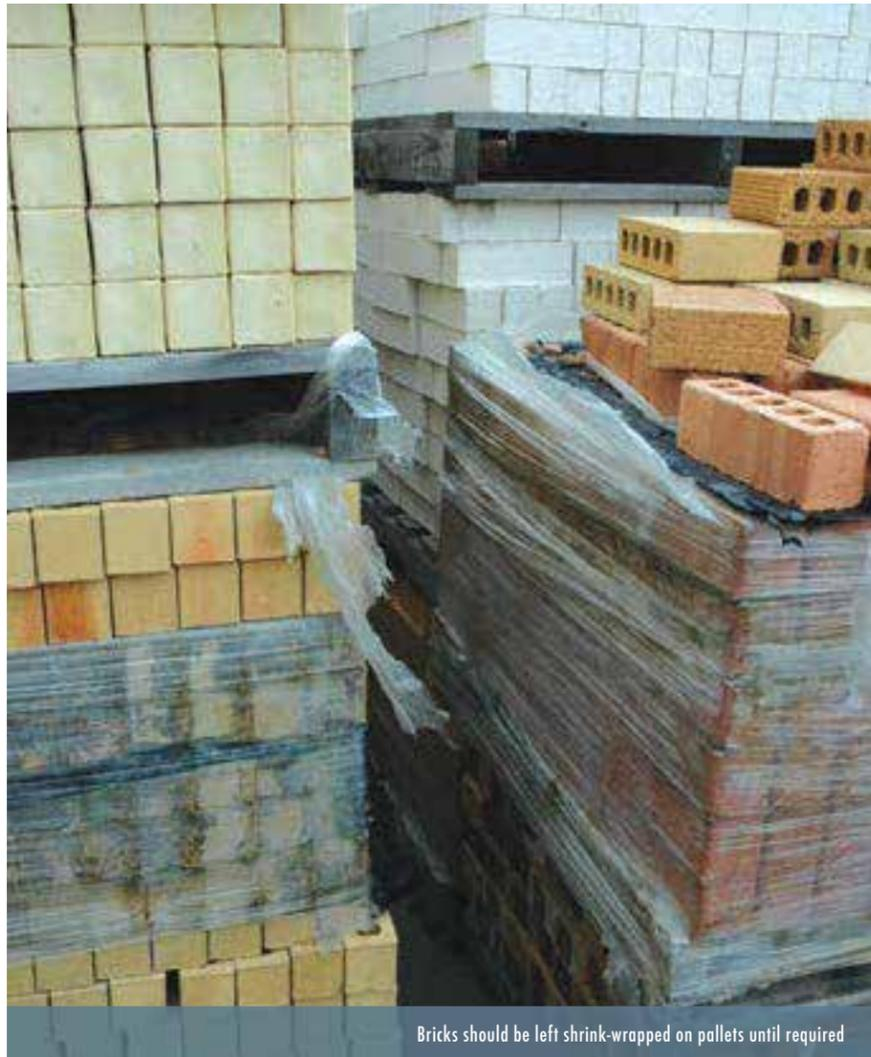
Bricks should be left shrink-wrapped on pallets until required
