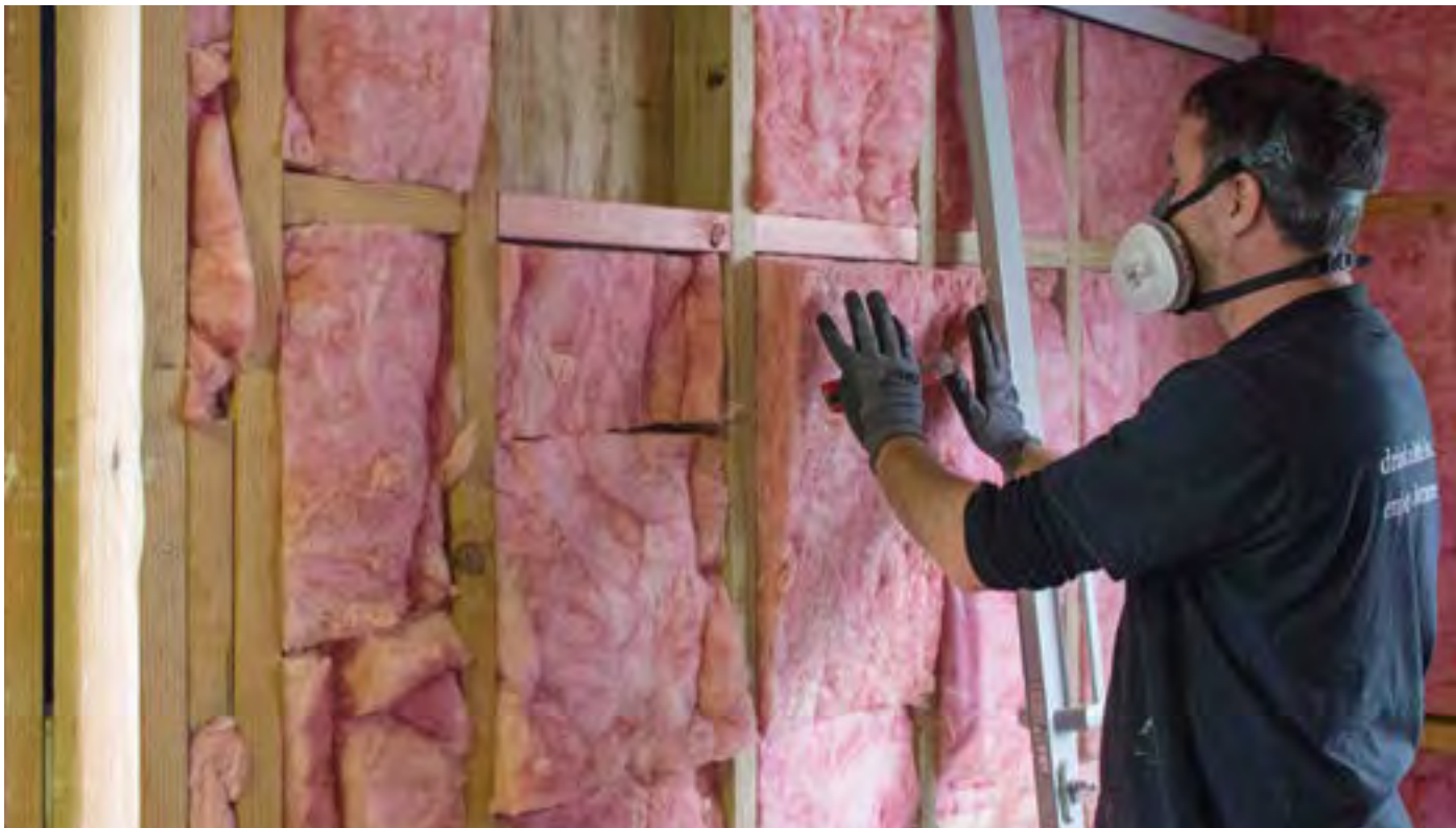
If linings or claddings need to be replaced, it is a good opportunity to install insulation at the same time. Remember, a building consent is required to retrofit insulation into existing walls
