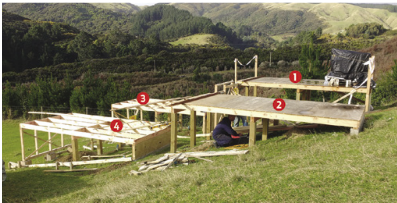
Test foundations being built – NZS 3604:2011 floors 1 and 2 on the right and pre-1960 floors 3 and 4 on left (Figure 2)
