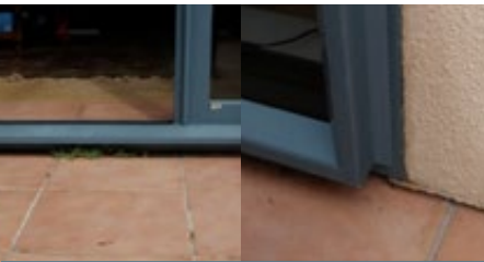
Stucco plaster cladding and joinery close to a tiled deck. Joinery installation issues at the jamb. Minimal threshold separation allows water uptake into the uncoated, porous bottom edge of the stucco plaster. Maintenance difficulties.
