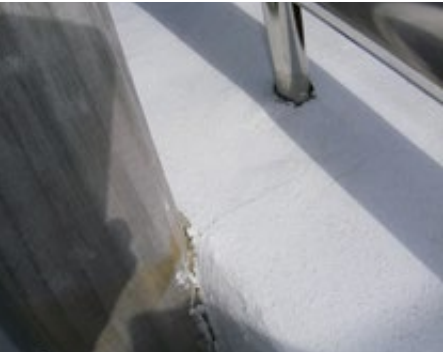
No kick-out or diverter provision at the bottom end of the apron junction to a fibre-cement cladding. Destructive testing confirms water ingress and timber damage.
