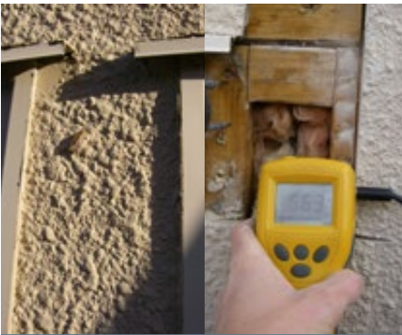
Texture-coated fibre-cement cladding. Window head flashings without stop-ends or other means of preventing water ingress. Coating and cladding sheets are in contact with the shoulder of the flashing which allows water uptake to the cladding edges by capillary action. Timber testing reveals visible water staining and a very high moisture reading. No evidence of proprietary waterproofing systems installation to window perimeter.
