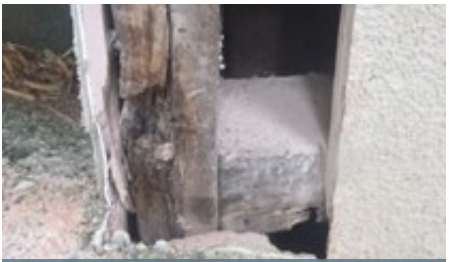
A fibre-cement clad timber-framed column and built-up paving resulting in significant damage.
