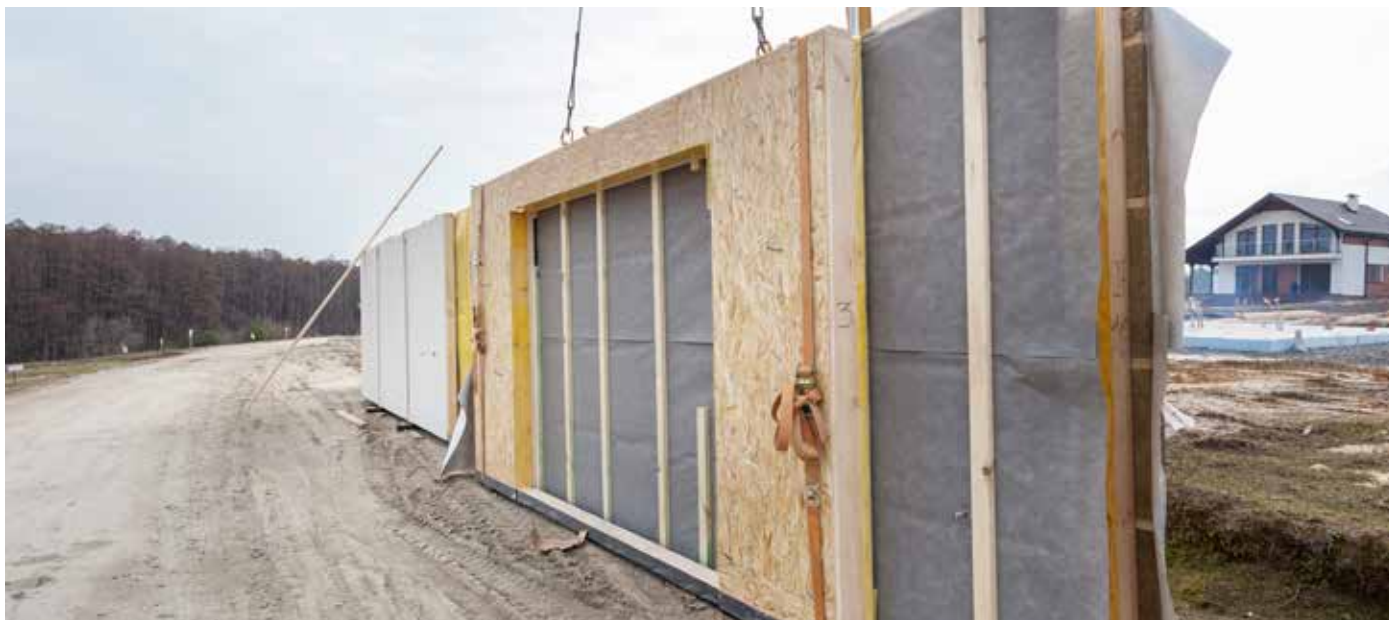
Structural insulated panels are becoming more popular for home building
